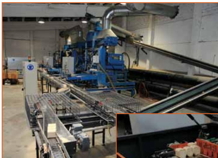
The wood briquettes are fully automatically transported from the presses to the packaging area on conveyor bands
